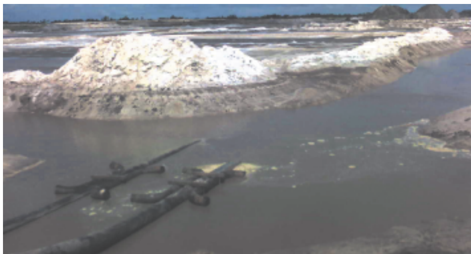
FIGURE 6: Construction Site Stormwater Run-Off Pump Station Inlet (July 28, 2008)
