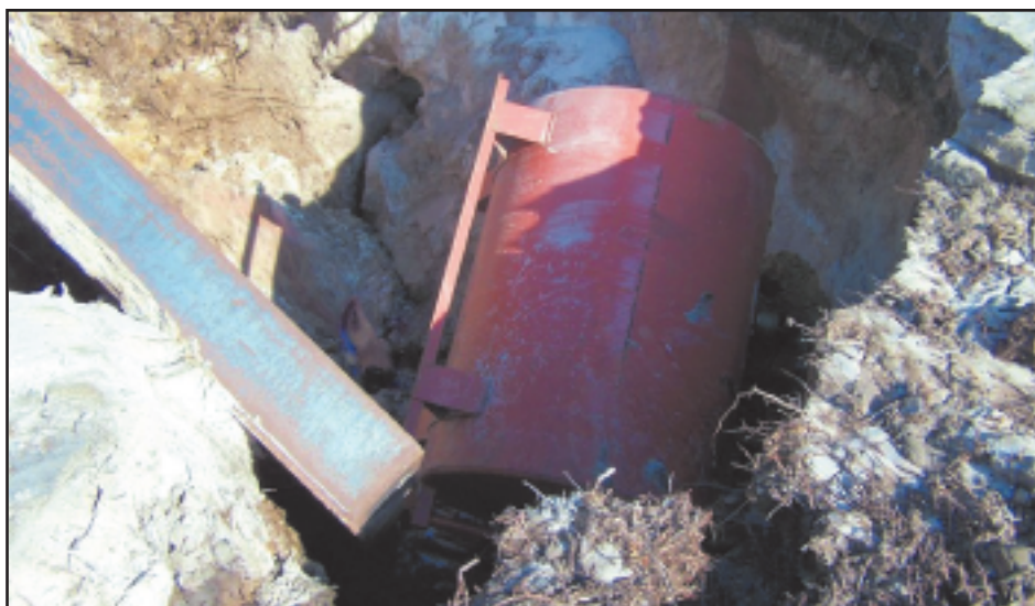
FIGURE 17: Diesel Spill Storage Tank Lying at Bottom of Erosion Gully
